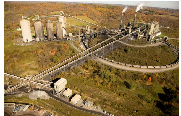
Figure 12 - Coal conveyor system and storage silos at CONSOL Energy's Bailey Central Preparation Plant
