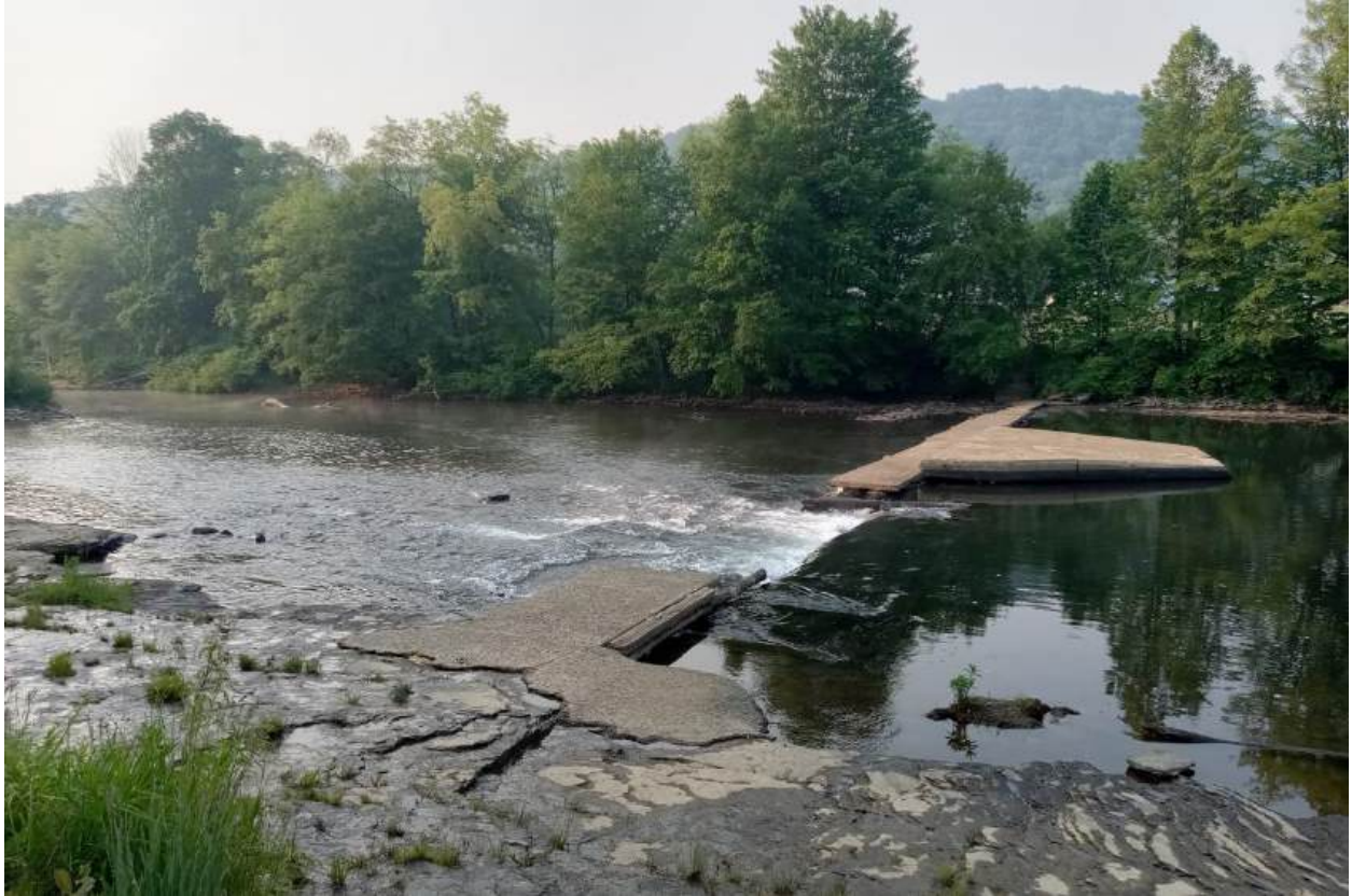
Figure 18: The failing low head dam is the subject of a conceptual design for removal and replacement with a whitewater structure.
