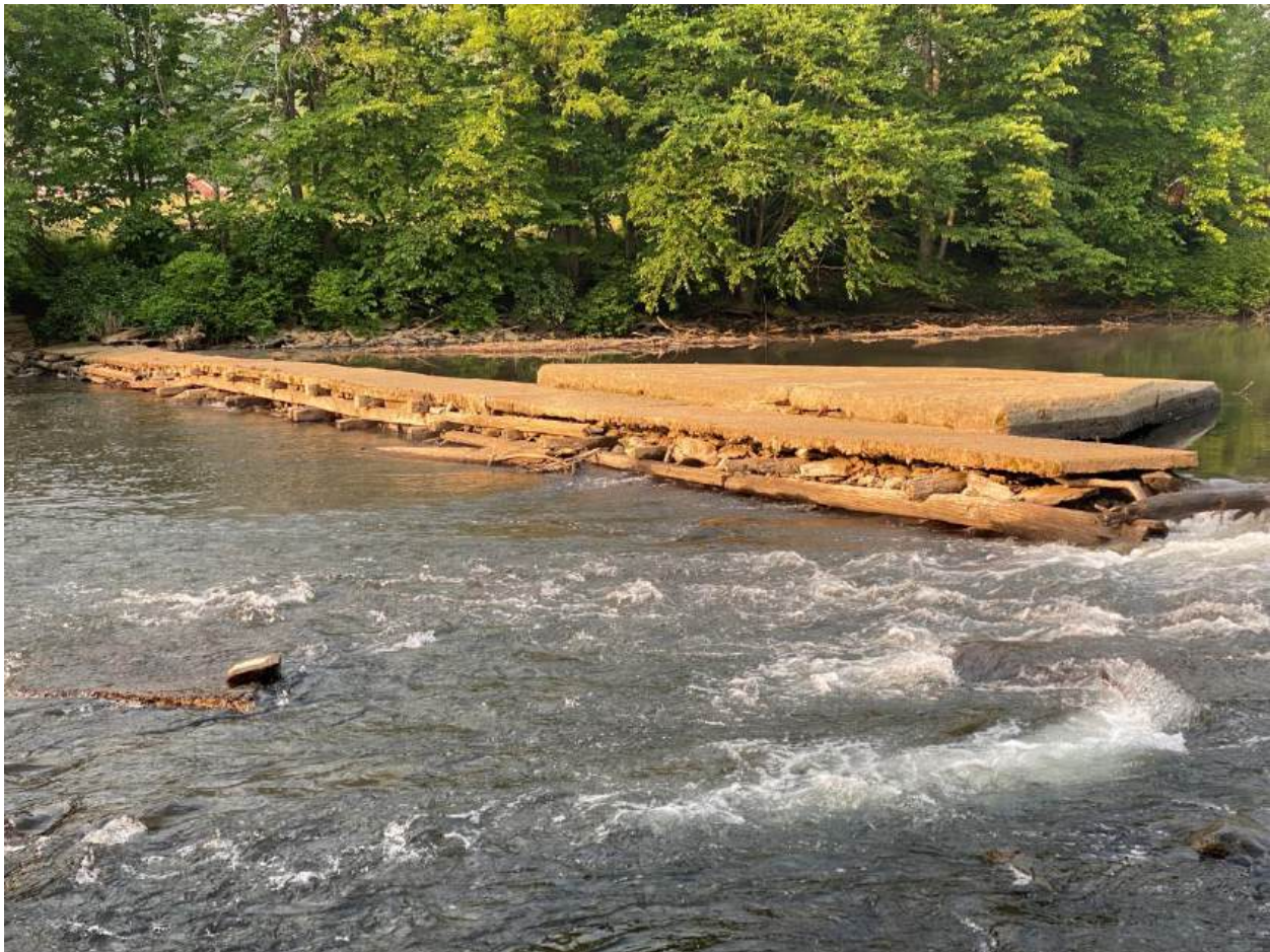
Figure 42: The Existing Dam has not been repaired since its most recent failure, which occurred sometime between 2013-2015. The dam appears to be constructed of timber and rock with a concrete layer. Given the current condition and construction of the dam, it is unlikely that repairing the dam will serve as a sustainable solution that would meet the community's needs.
