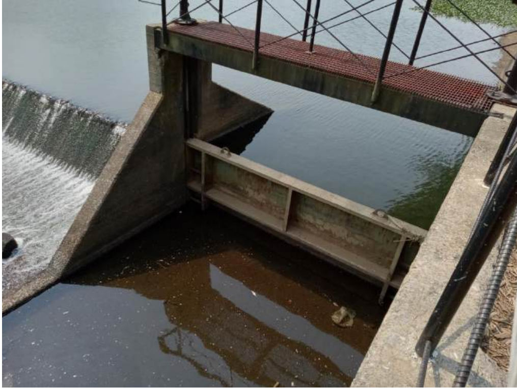
Figure 32: The river left side of the dam features a manually operated sluice gate within a concrete structure.
