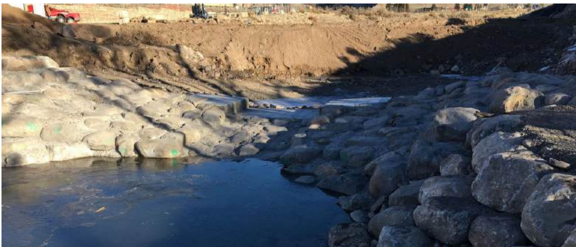
Figure 38: This structure, dewatered and under construction, shows what S 2 O designed whitewater structures look like under the water surface - the center low flow notch channelizes the river to get the most out of available flow, and interstitial spaces between boulders aid in fish passage through the structure at all water levels. The next "stair step" up is to accommodate medium flows, and higher flows rise along the grouted boulder slopes of the structure towards the banks.
