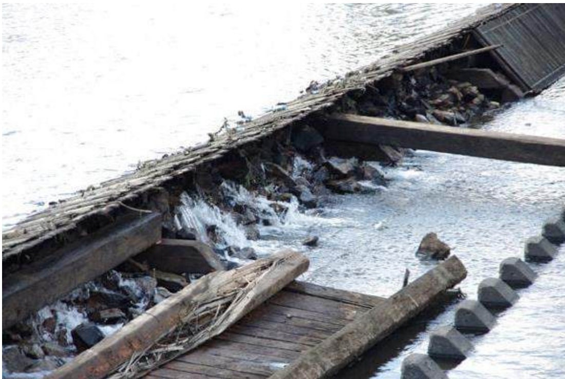
Figure 45: In the September 2016 failure of the Raftsman Dam, a 60-foot section of the dam broke off. The dam appears to be timber framing filled with rocks and additional timber, with a concrete pad below. Photo from Courier-Express Article.
